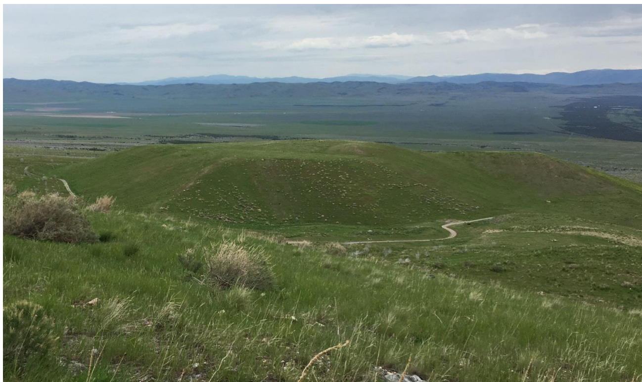
Figure 4.3 View of the Reclaimed Black Pine Mine Heap-Leach Pad, Looking East (from Liberty Gold, 2017)
